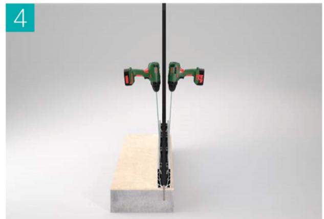
Adjust the inclination of the glass using the screws on the clamps with a 5/32" (4 mm) hex driver and tighten.
